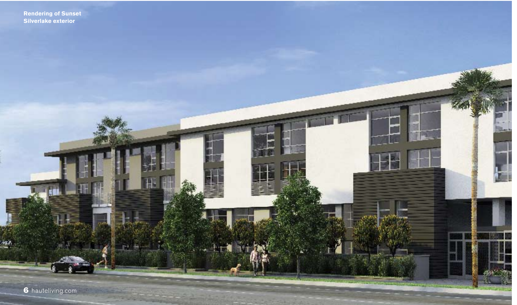
The rooftop at Broadway Hollywood
